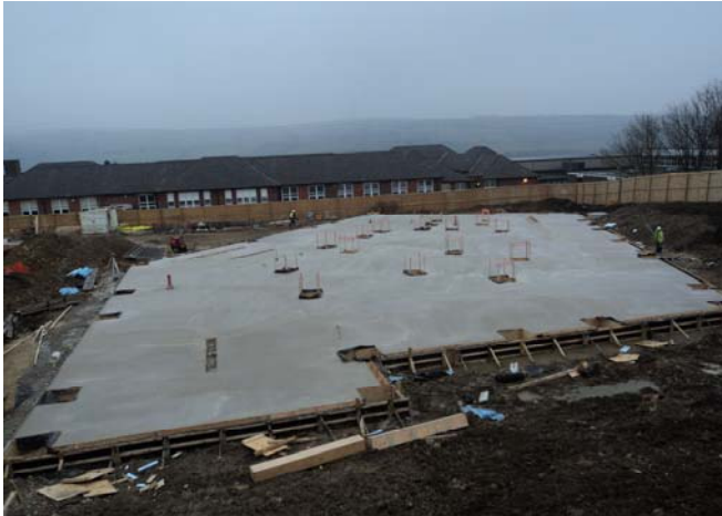
Above shows the ground floor slab which is now completed.
