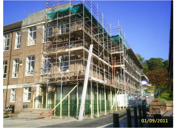
Scaffolding for the New Roof to Building A1
