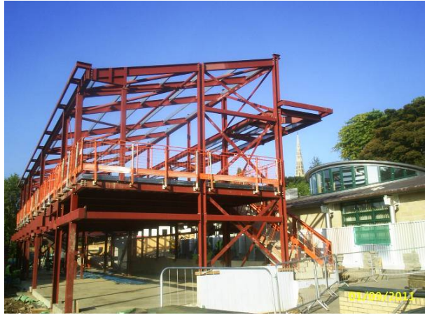
New Building Steelwork
