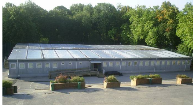
The Modular Building Housing Temporary Classrooms.
