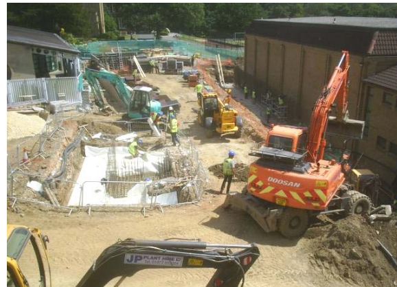
Foundation Works to New Building
