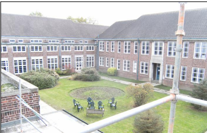
One of the existing courtyards – Tidy, safe and usable once more
