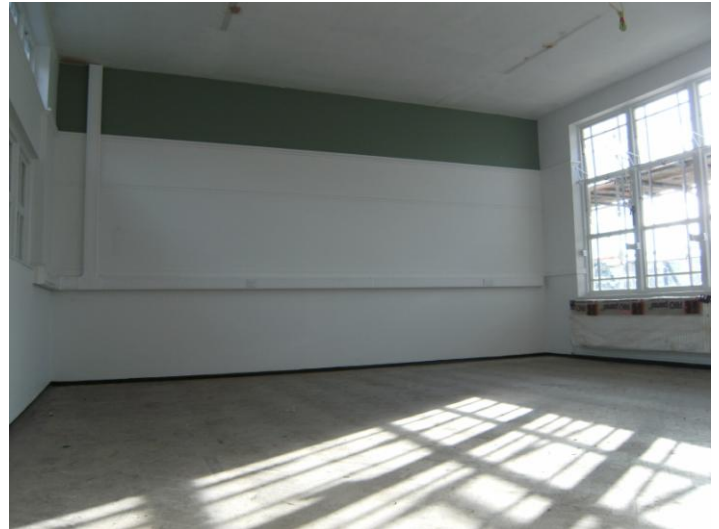
The Sample room – Getting ready for the final fittings
