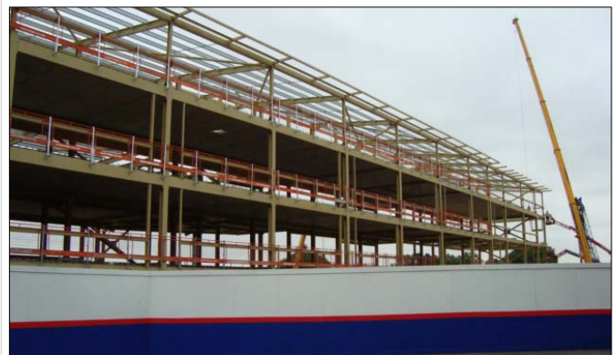
The steel currently erected at Forge Valley School
