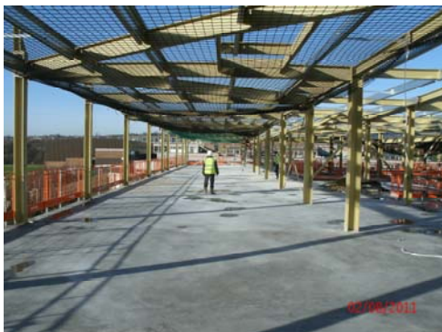
Block 1 - Floor Slab Construction
