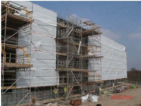
Block 1 - Scaffolding to South Elevation
