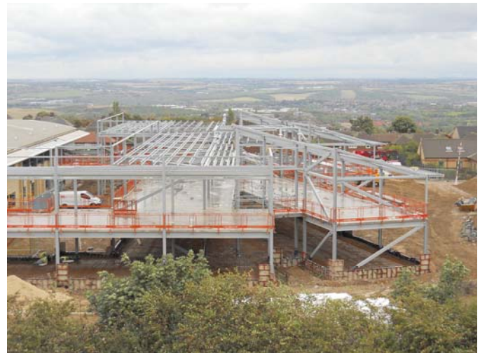
The Steel Frame takes shape
