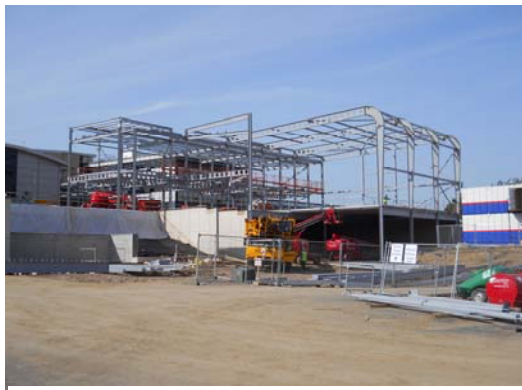
The Steel frame installation continues
