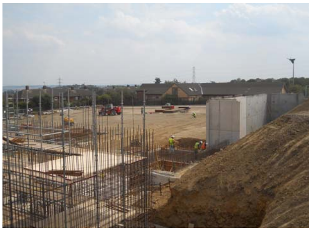
Extensive Concrete Foundation works progressing
