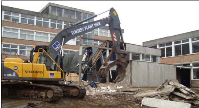
Demolition of the VOTEC Centre
