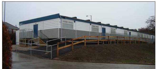
Temporary classrooms erected for the students of Myers Grove
