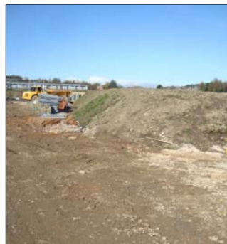
Topsoil stored ready to be reused on site
