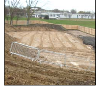
The excavation works for the new Sports Block
